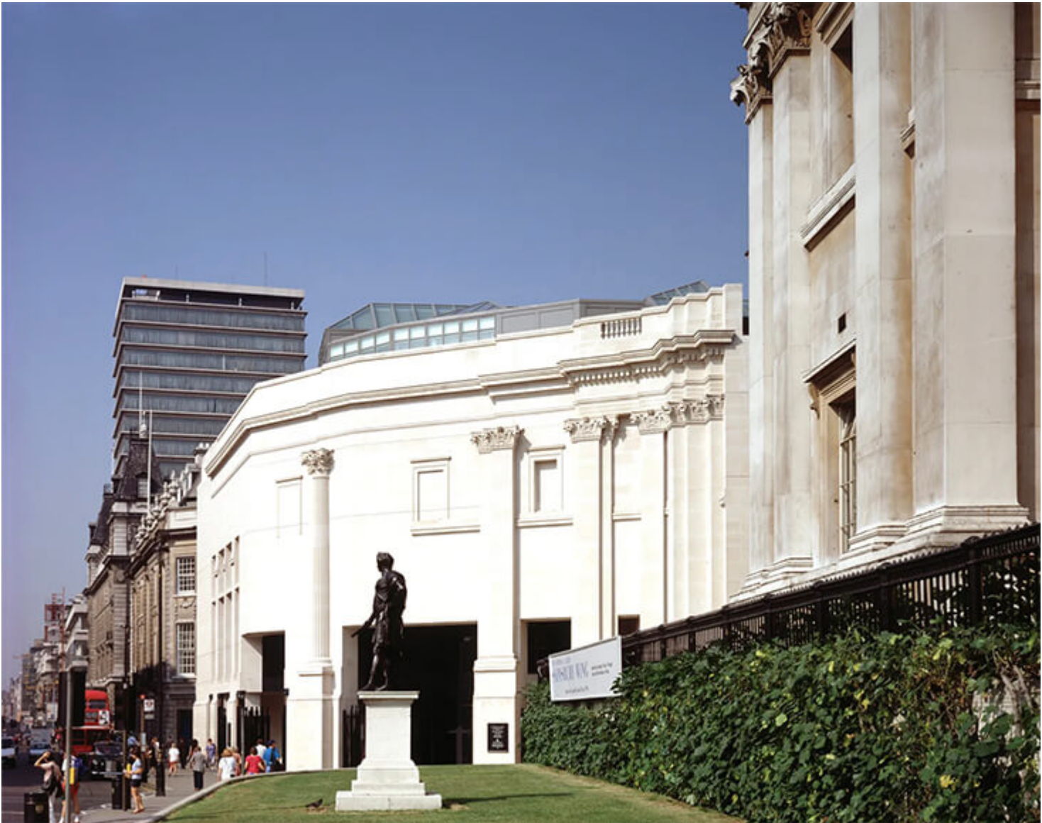
Venturi Scott Brown & Associates Sainsbury Wing of the National Gallery, London, 1991, featuring reduced and simplified Neoclassical columns
