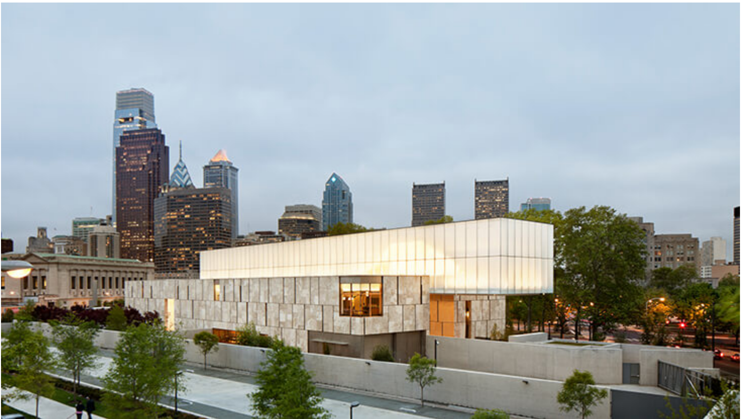
The Barnes Foundation designed by Tod Williams Billie Tsien Architects
